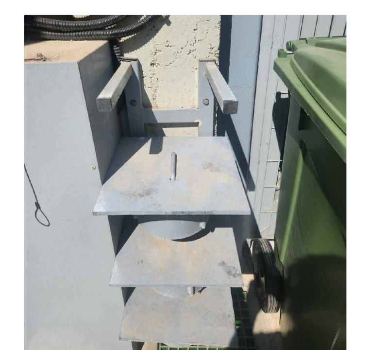
BARRIER CYLINDER COVER'S STORAGE FACILITY FOR 4 COVERS
